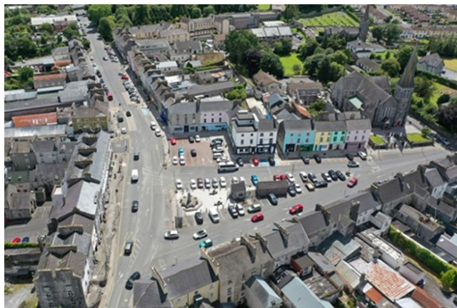
Existing condition at R458 to R460 junction at Gort Market Square
